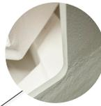
All structural bulkheads and reinforcement are glued and laminated to the hull and deck.
